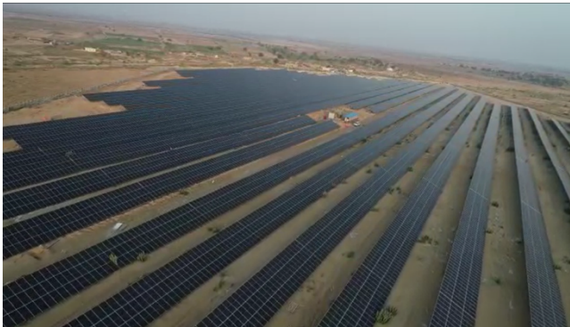
EPC for BOS of 300MW Ground mounted Solar Power Project at Rajasthan, India
