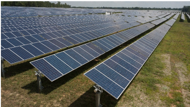
EPC of 40MW Ground mounted Solar Power Project at Rajasthan, India
