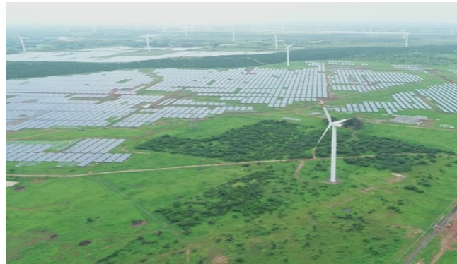
EPC for 100MW (AC) Ground Mounted Solar Power Project at Tamil Nadu, India
