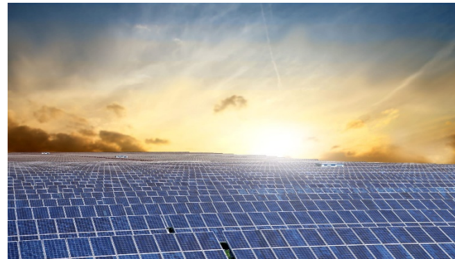
EPC for 45MW Ground Mounted Solar Power Project at UP, India
